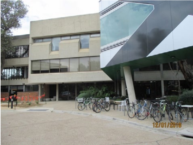
View of the R.N Robertson Building
